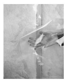
This product can be used in place of traditional vapor retarders with unfaced fiber glass insulation to provide an insulation system that is ideal in some of the more severe climate condition areas in terms of both temperature and humidity.
